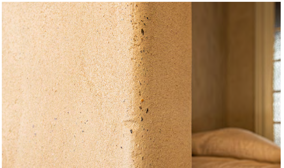
Sponging results into a homogenous surface. For Léém Clay Plaster, which has a bigger granulometry, gravels may become more visible depending on the moment and intensity of sponging
