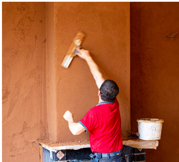
Levelling the surface of the Léém Plaster with a smoothing trowel
