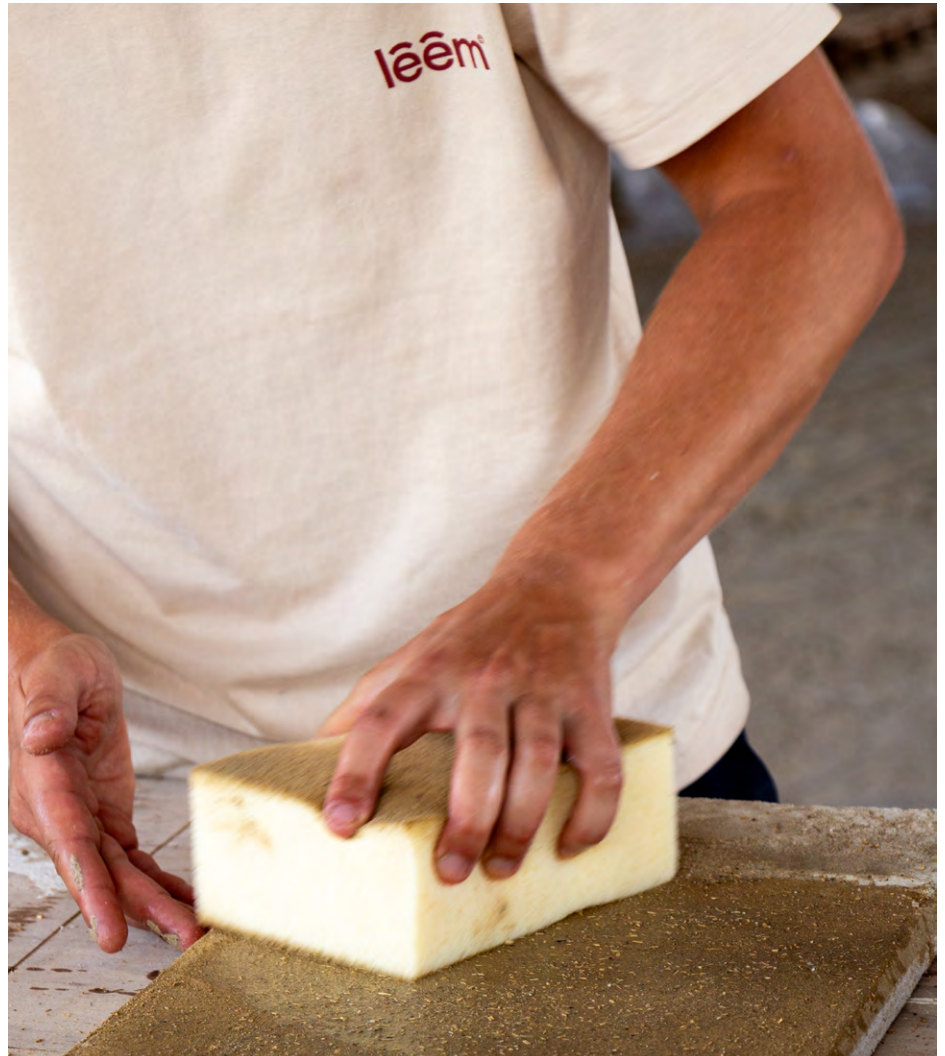
Clay plaster with a large amount of straw fibre
