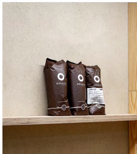
Léém Clay Plaster finely sponged in the office building of the order of architects, Brussels
