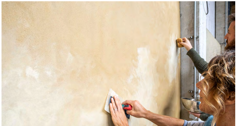
Using a plastic flexible trowel allows to reach a polished smooth surface
