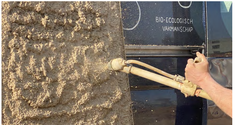
Léem Clay plaster applied with a spraying machine
