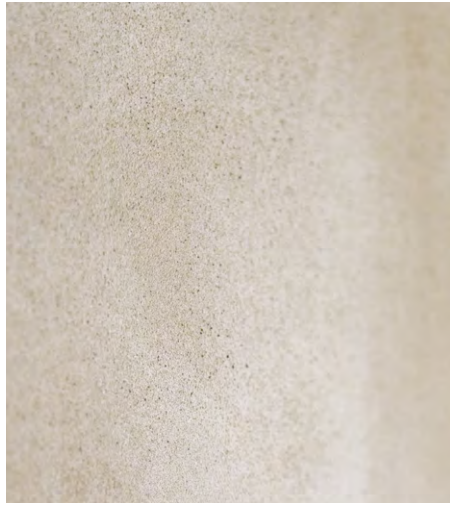
Final result of a smoothly polished Léém Clay Finish
