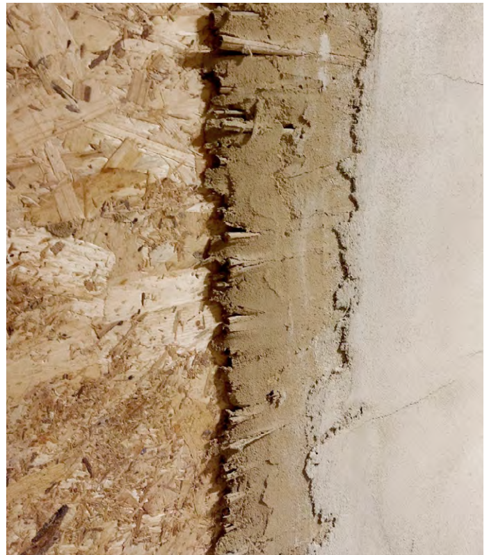
OSB panels with reed lath stapled on it. The reed lath should be covered sufficiently (more than on this image) to create a homogenous base coat and avoid cracks
