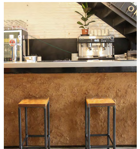
Léém Clay Plaster applied and finished purposely in a very rough way. Bar of Ancienne Belgique, Brussels
