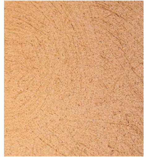
Pronounced texture of a rough wood float
