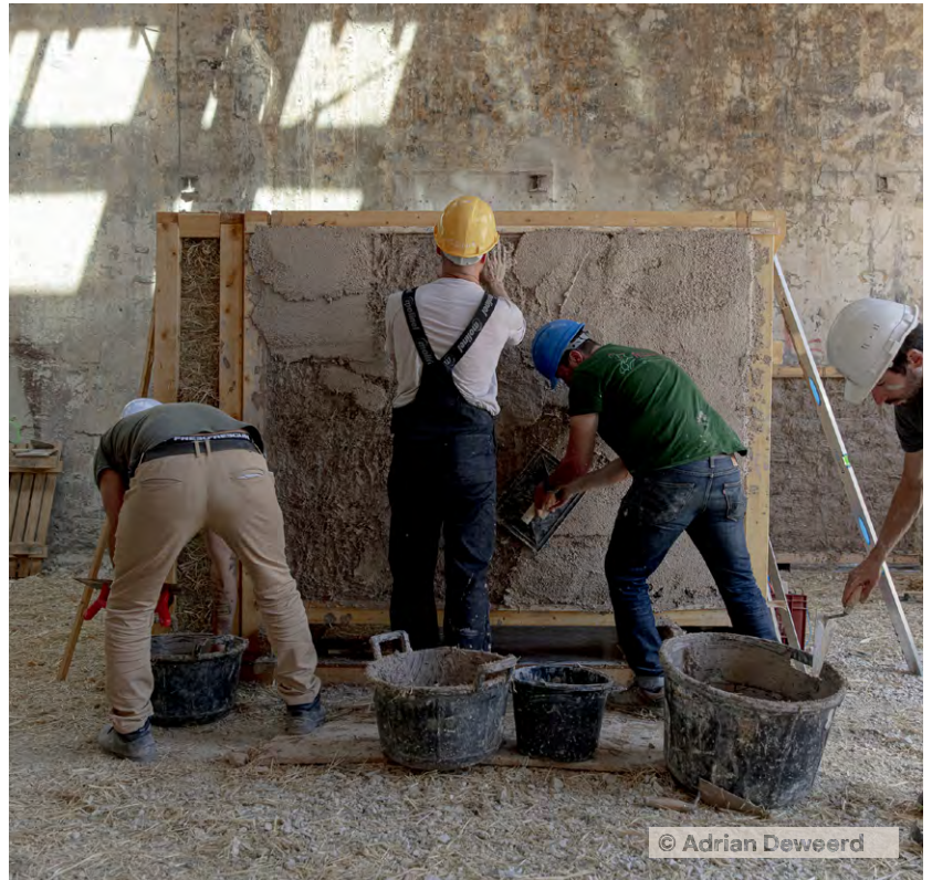
Prototype of clay plaster on straw bales
