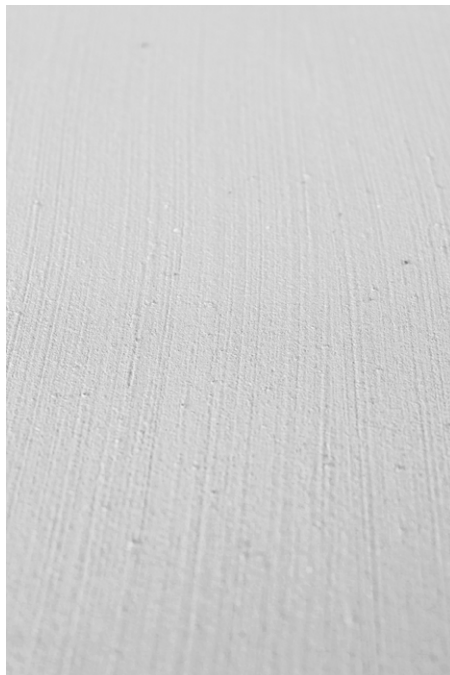
The Léém Clay Paint has been applied with rough brush strokes, these create a textured result
