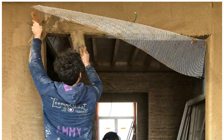
Léém Flax Reinforcement Mesh embedded in the base coat, covering the lintel
