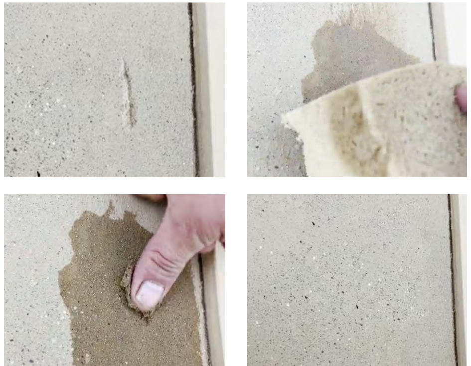
Reparation process of a scar in the Léém Plaster
