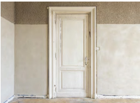
A distance of 5cm is kept between the floor and the Léém Clay Plaster
