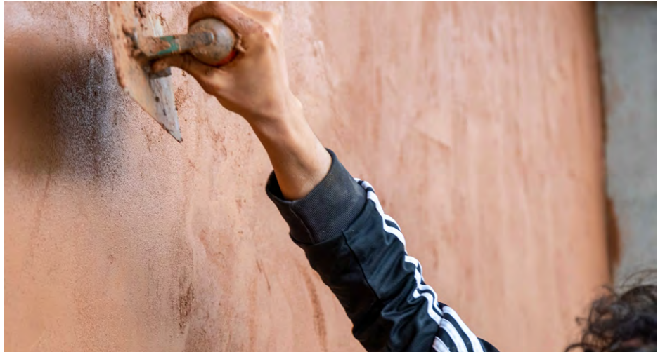
Léem Clay plaster applied manually with a trowel
