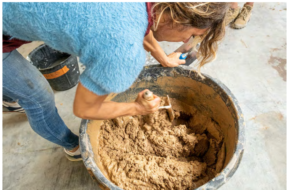
Preparation of Léém Clay Plaster
